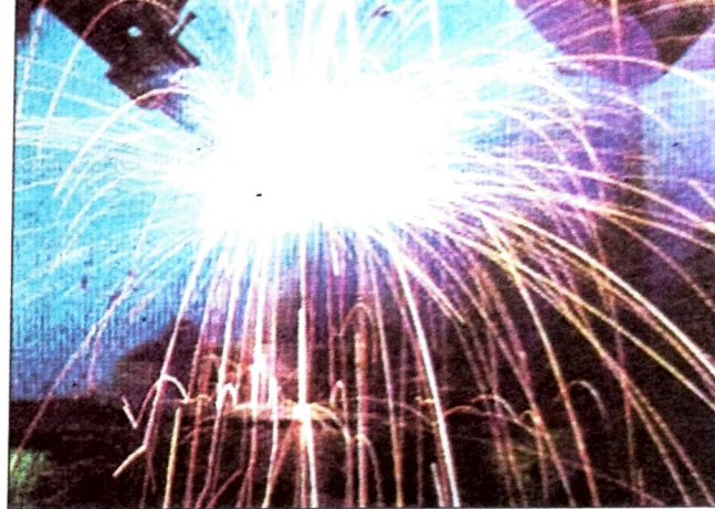
Electric arc welding
